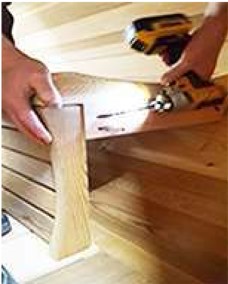
If the electric heater option was chosen, screw the angled bench support to the short front enclosure using 2 ½" (64mm) screws in the pre drilled holes.
